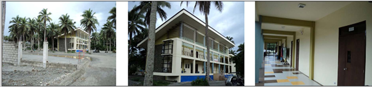
SHS Extension Campus, Baler
